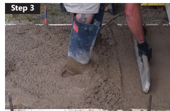
Step 3 PCC Leveling
