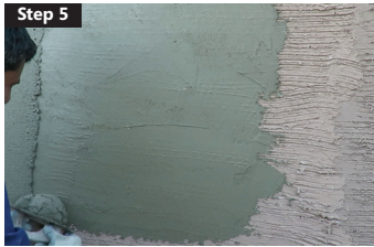
Step 5 Load material as plaster for stamping in required thickness
