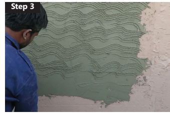
Step 3 Draw scratch coat
