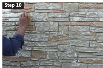
Step 10 Applying colours randomly
