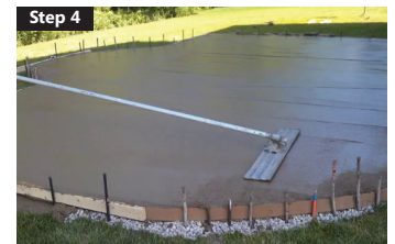
Step 4 PCC finishing
