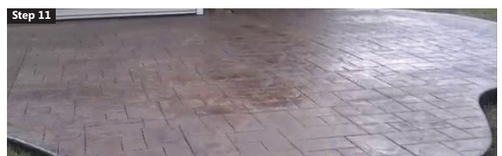
Step 11 Final view after top coating
