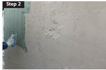
Step 2 Load thin material on wall
