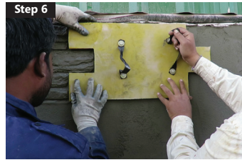
Step 6 Stamping Dye in interlocking manner
