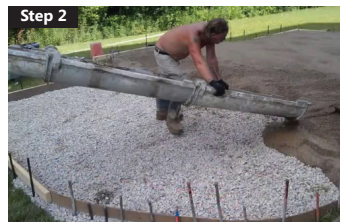
Step 2 PCC flooring
