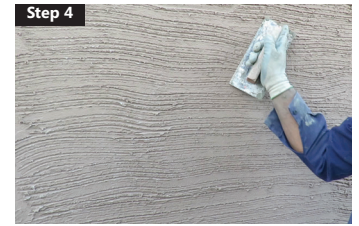
Step 4 Remove excess material
