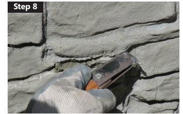
Step 8 Scrapping excess material
